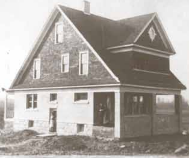
Frank and Mary's new home, completed just in time for Thanksgiving dinner 1914. The home later served as FEN's office until 2001.
